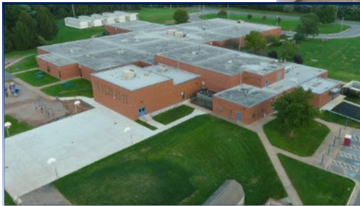
Mountain View ES – Renovation
