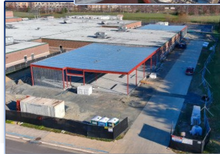
Gainesville MS – 11-classroom addition
