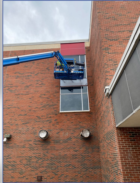
Unity Reed High School Fenestration Improvements
