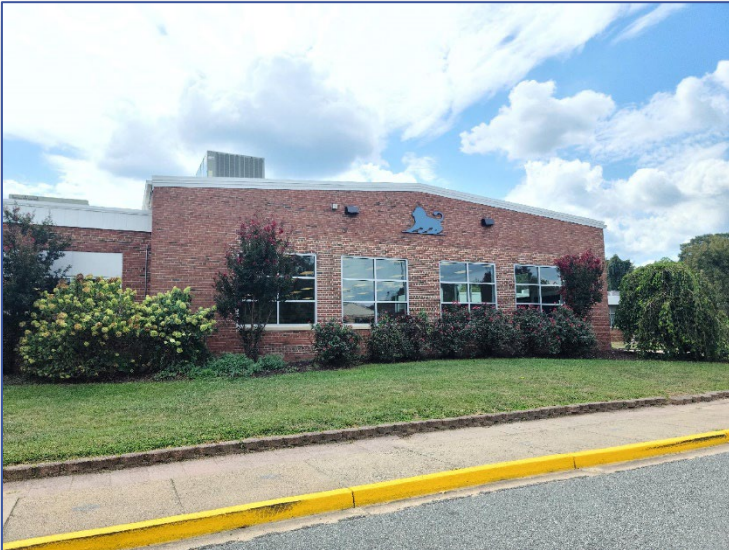
Graham Park Middle School Fenestration Improvements
