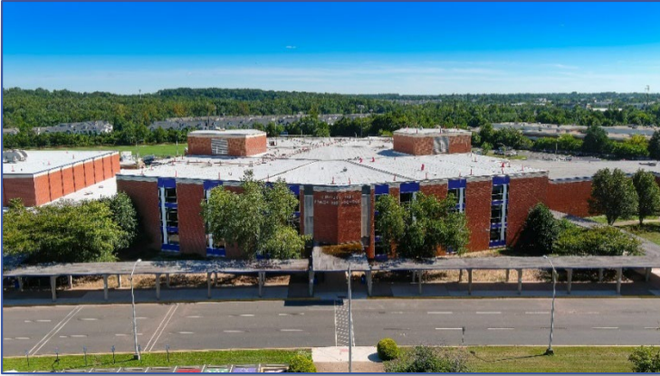
Osborn Park High School Fenestration Improvements
