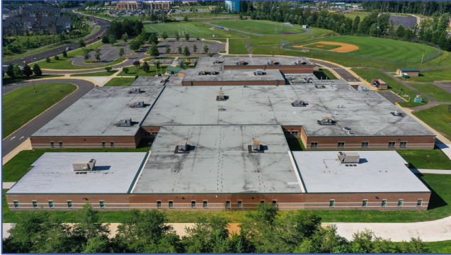
Gainesville Middle School 11-Classroom Addition
