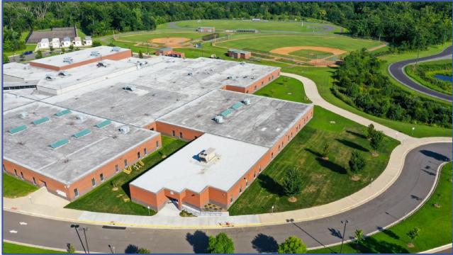
Reagan Middle School 6-Classroom Addition
